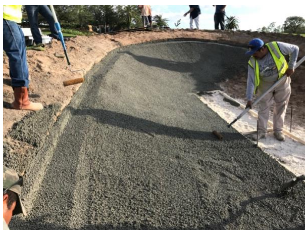
Creation of Capillary Concrete Edge
