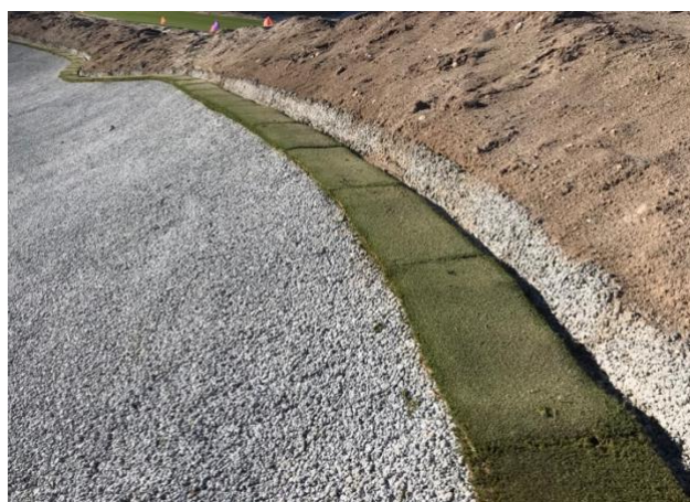
Profile, 1st layers of EcoBunker done, 2 layers of natural turf to go
